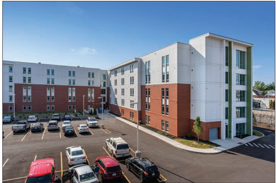
Fairfield Landing, a 197-unit housing complex, along with Stephen J. Kopp Hall, opened in August 2019.
